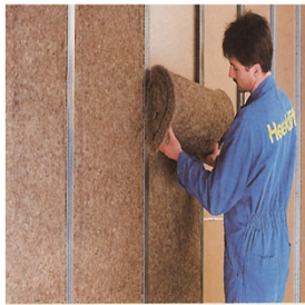
Wool fleece into internal wall
