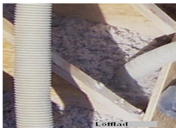
Loose insulation blown into cavities (Cellulose fibres from Isofloc)
