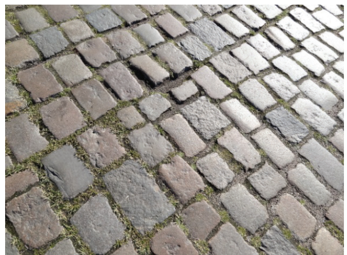
Figure 39: Cobble stones in city centre Source: Ziel 2012
