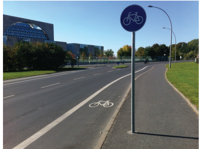
Figure 10: Cycle lane outside built-up area, Berlin (Germany) Source: Müller 2011
