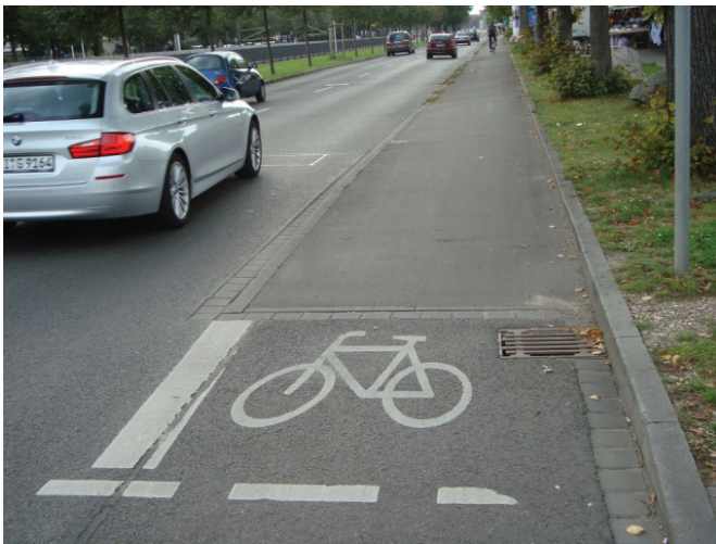
Figure 18: Parallel cycle track, intersection area, Leipzig (Germany) Source: Rudolph 2011
