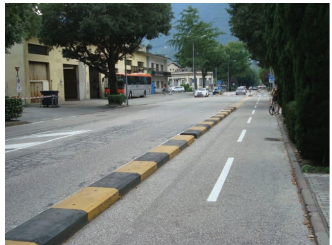
Figure 24: Independent cycle track physically separated from motor traffic, Bolzano (Italy) Source: Rudolph 2011
