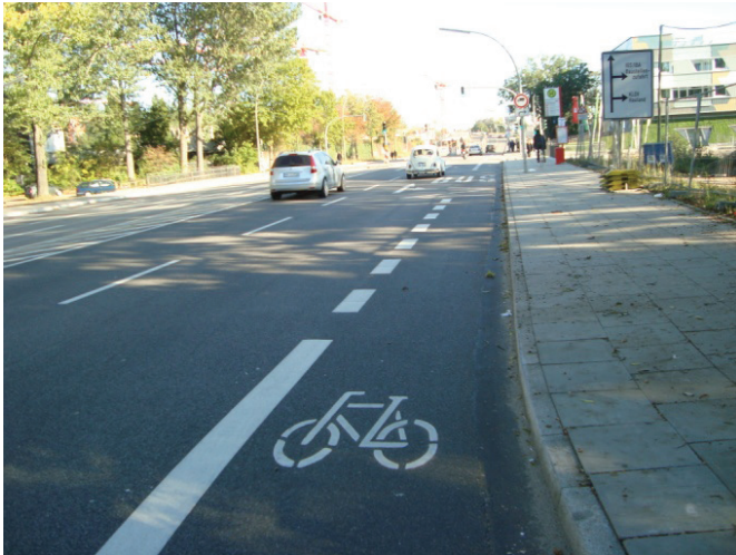
Figure 9: Cycle lane outside built-up area, bus stop area, Leipzig (Germany) Source: Rudolph 2011
