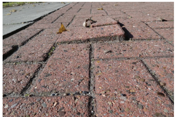
Figure 54: Poorly installed tiles, Hamburg (Germany) Source: Rudolph 2011
