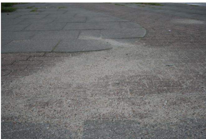
Figure 63: Removing grit after winter service, Hamburg (Germany) Source: Rudolph 2011
