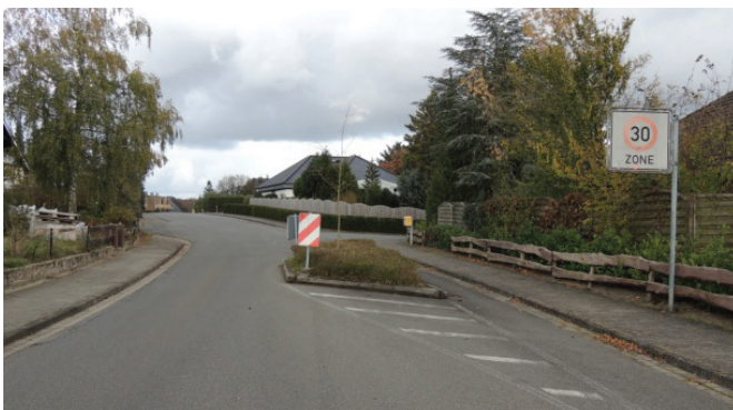
Figure 37: Gateway to a 30 km/h-Zone Source: Fricke 2012
