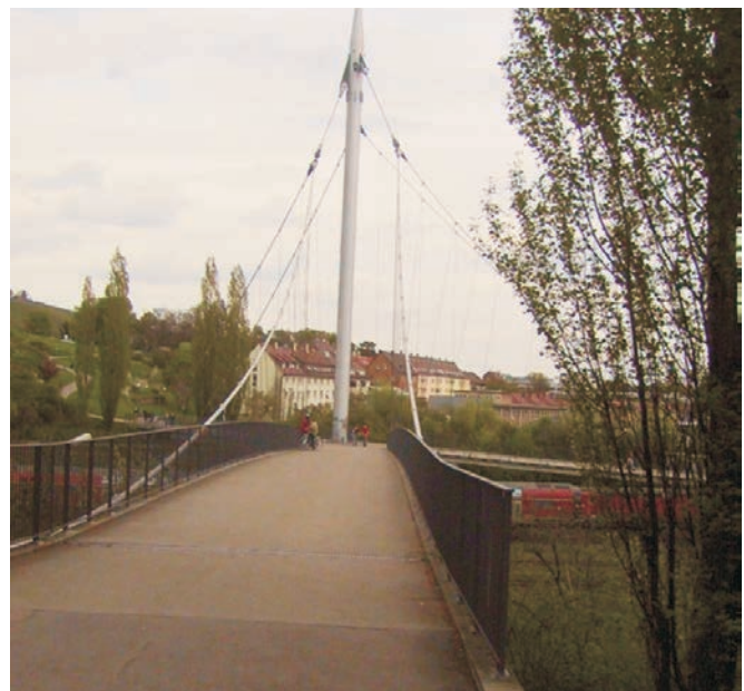
Figure 82: Cycling bridge over railroad, Stuttgart (Germany)
