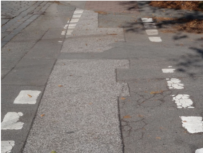
Figure 62: Poorly maintained markings and surface, Hamburg (Germany) Source: Rudolph 2011
