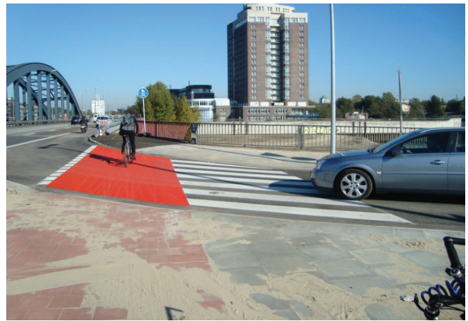
Figure 33: Cycle track crossing road, Hamburg (Germany) Source: Rudolph 2011
