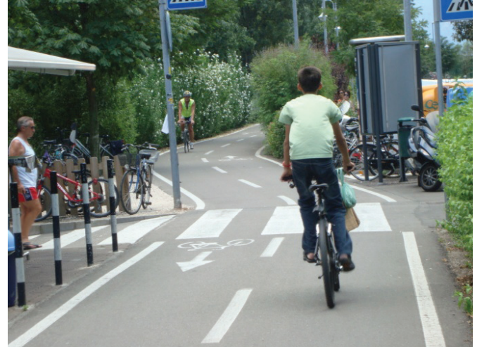
Figure 26: Independent cycle track, Bolzano (Italy) Source: Rudolph 2011
