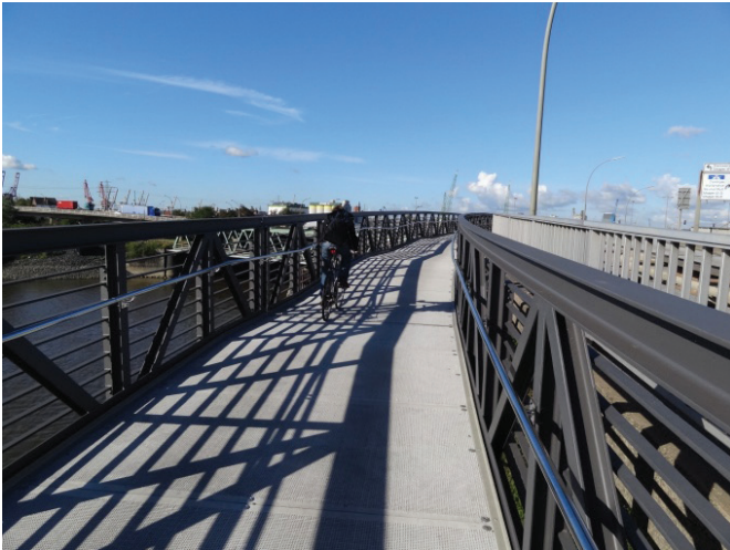
Figure 83: Bicycle bridge, Hamburg (Germany) Source: Müller 2011
