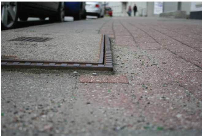
Figure 71: Manhole with edge elevated up to 2,5 cm above pavement, Hamburg (Germany) Source: Rudolph 2011
