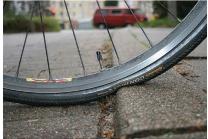
Figure 60: Kerb stone concrete showing impact to wheel even with rounded edge, Hamburg (Germany) Source: Rudolph 2011
