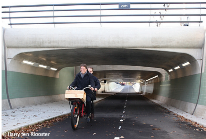
Figure 81: Bicycle tunnel, Zwolle (Netherlands)
