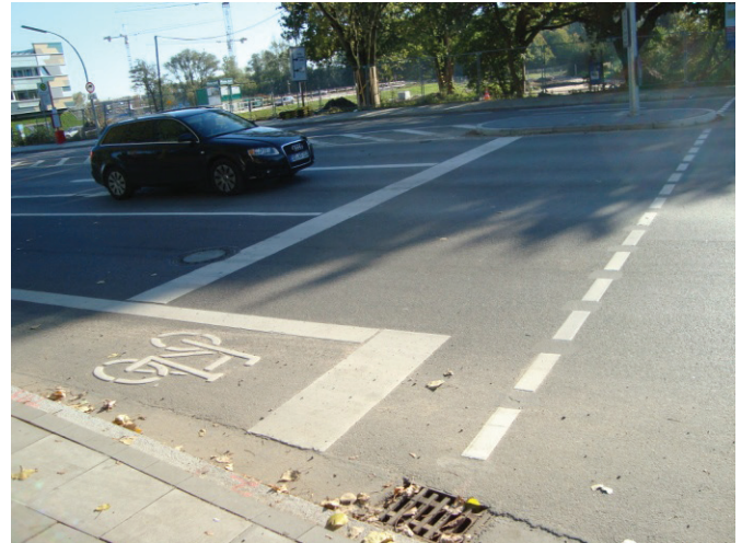
Figure 84: Advanced stop line, Hamburg (Germany) Source: Rudolph 2011
