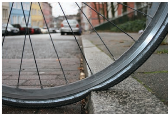
Figure 59: Kerb stone granite showing impact to wheel, Hamburg (Germany) Source: Rudolph 2011
