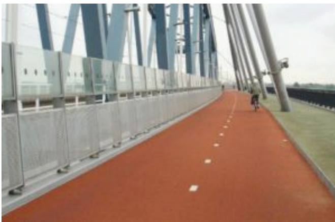
Figure 93: Bicycle highway constructed in the Netherlands Source: fietsen.123.nl
