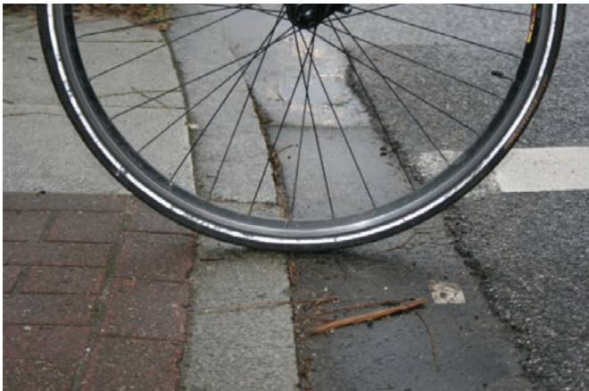
Figure 58: Kerb stone granite with even transition between cycle track and road pavement, Hamburg (Germany) Source: Rudolph 2011
