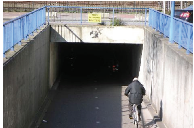
Figure 79: Tunnel not attractive: dark, end of tunnel not visible, relatively small (Netherlands) Source: Noordholland Dagblad
