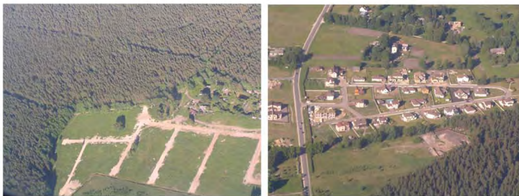
Figure 0: Building activities in the green belts round the cities (Photo: Dirk Schröder-Brandt).
