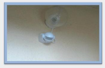
If during the day time, it is bright enough in the staircase, a motion sensor with the so called "twilight switch" is required, letting the unit to run only when the light is falling.
