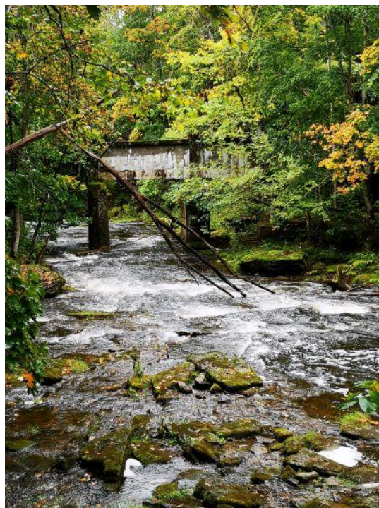
Photo 5. Remains of Nõmmeveski hydropower station (S. Oisalu)
